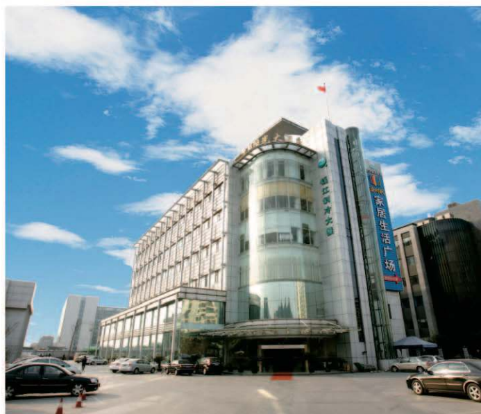
The company headquarters
